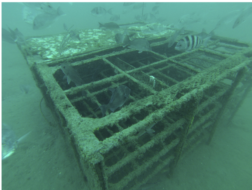
Fig. 1. Steel cage artificial reef site used in the present study. Dimensions of reef are 2.5 m length x 2.4 m width x 1.3 m height.
