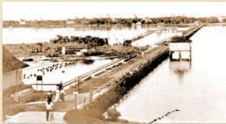
THE SOUTH BRIDGE WAS ONE OF THREE BRIDGES THAT LINKED DAYTONA WITH THE BEACHSIDE. BUILT IN THE 1890S, SOUTH BRIDGE WAS ALSO HOME TO DAYTONA'S JAIL WHICH WAS LOCATED IN THE MIDDLE OF THE RIVER.
