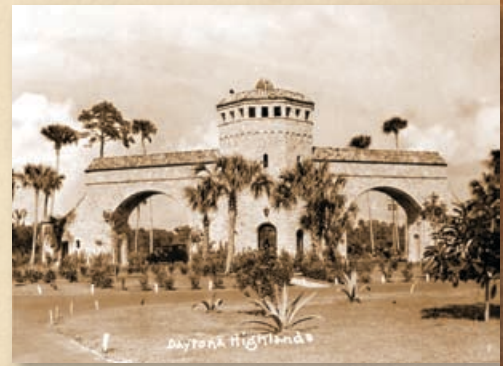
A PORTION OF THE OLD TERRAGONA ARCH THAT WELCOMED VISITORS TO THE DAYTONA HIGHLANDS SUBDIVISION IN 1925 CAN STILL BE SEEN ALONG INTERNATIONAL SPEEDWAY BLVD. TODAY.
