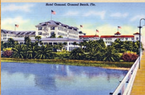
COMPLETED IN 1888, THE ORMOND HOTEL PAVED THE WAY FOR FUTURE RESORTS ALONG THE "WORLD'S MOST FAMOUS BEACH"
